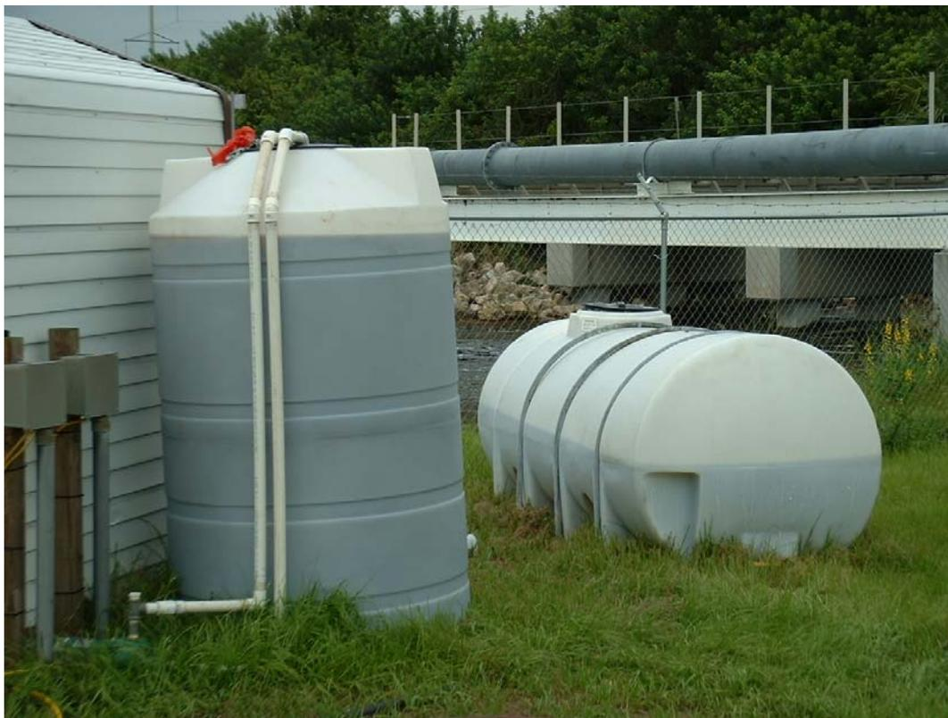
Figure 6-2. Storage Tanks for Alum and Polymer.
