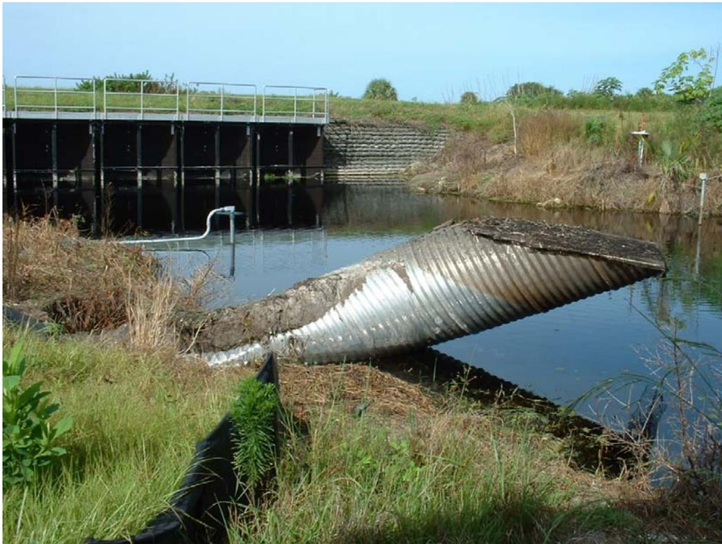
Figure 5-1. Dislodged Intake Pipe.
