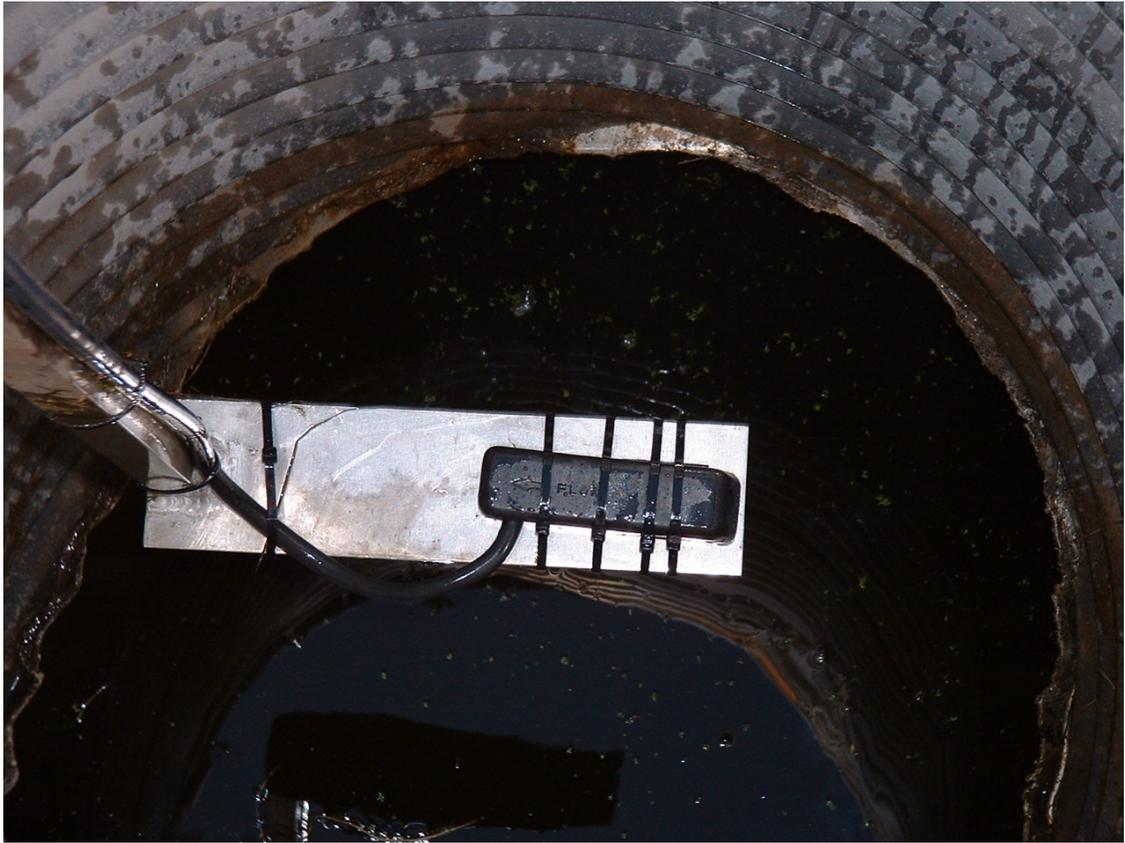
g. Area-velocity Probe Attached to Mounting Pole
