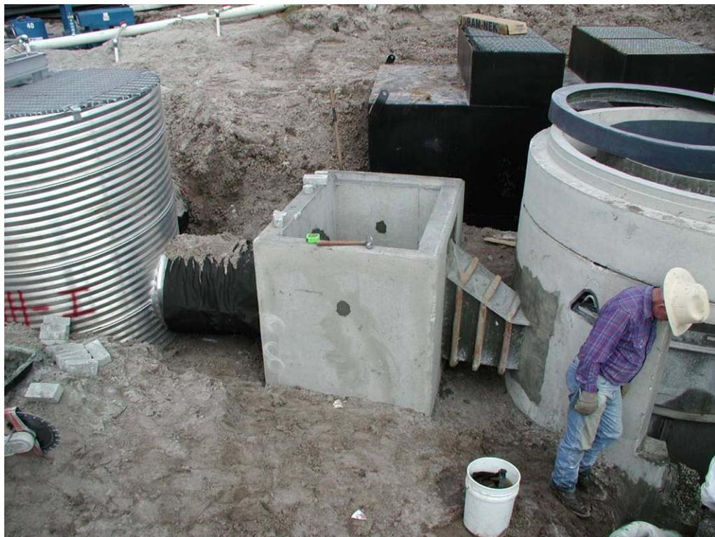
l. Connection Structure for CDS Unit
