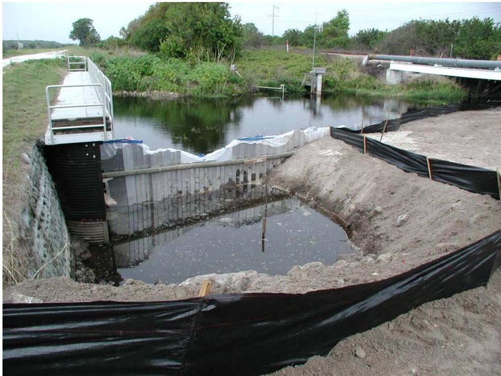
n. Installation of Sheet Pile for Isolating CDS and TST Outfall Pipes
